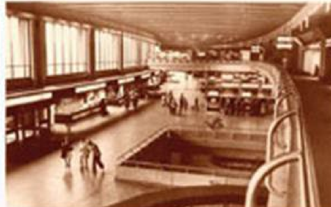
The departures level concourse features long open unobstructed areas and the openness of the design creates a visual link between the three main levels of the building. Paved concrete is a dominant feature throughout the interior of the terminal building.
