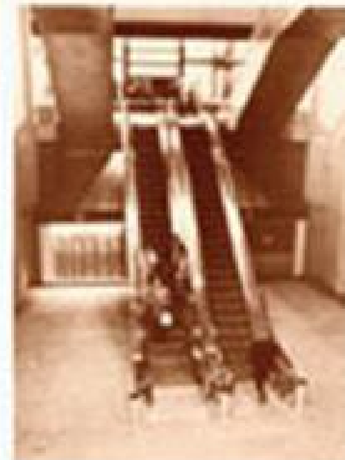
Three main escalators ensure efficient flow of traffic in the central portion while stair structures also conveniently located throughout the terminal.
