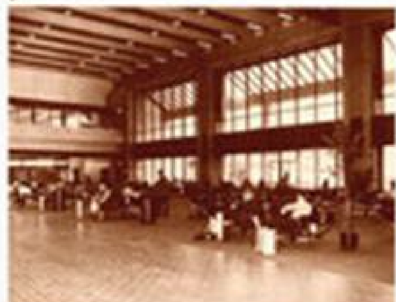
The drive-to-gate departure level providing area for ground service between the Cities of Calgary and Edmonton.
